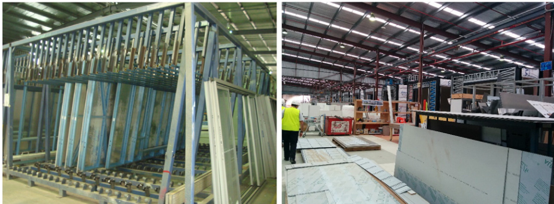
Fig. 1. Off-site construction plants in the two cases.
