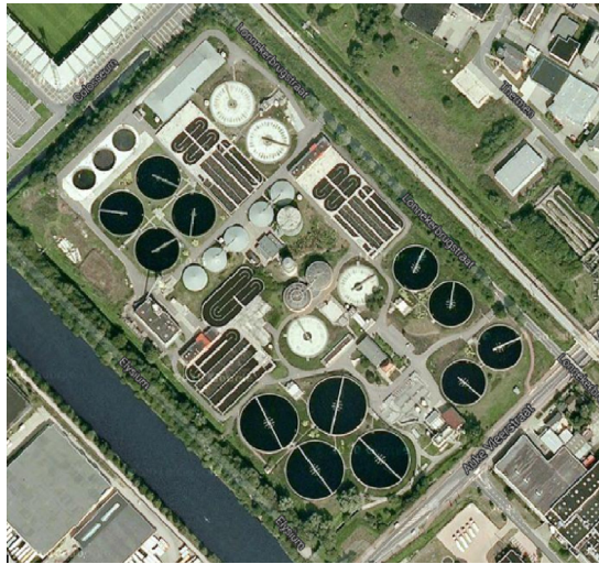
Fig. 1. A bird's eye view picture of the sewage treatment facility in Enschede, the Netherlands. The picture is retrieved using Google Maps.
