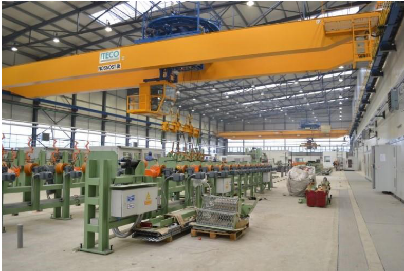
Fig. 1. Steel hall with a crane runway.
