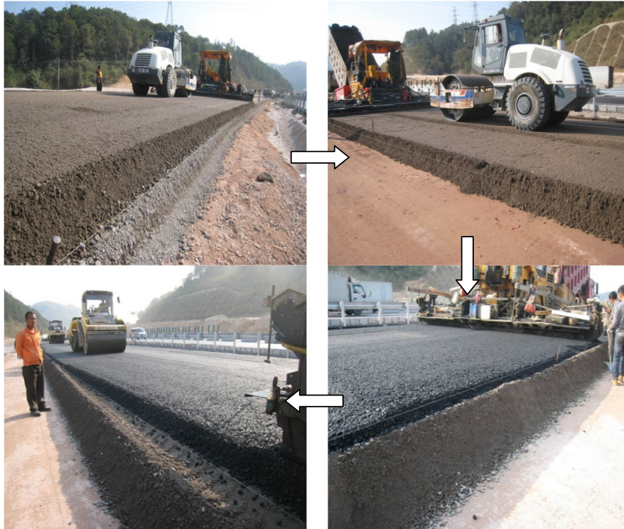
Fig. 2. Pavement construction process of CCM.
